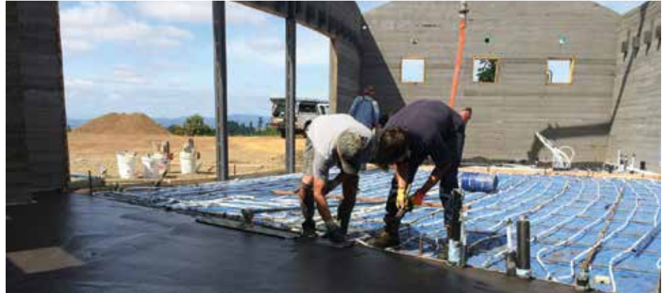
▲ Fairsing Vineyard uniquely designed tasting lounge utilizing a single heat source known as "Radiant" heating, enveloped with integral "Color" concrete completes the architecturally designed floor .
