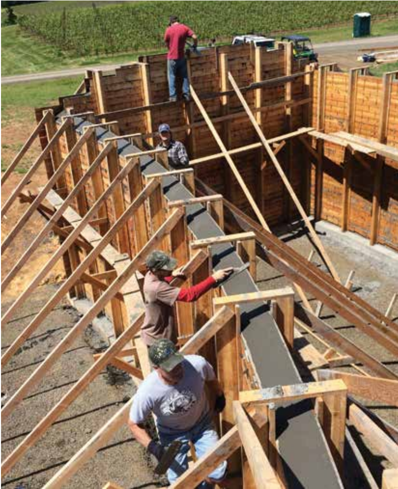
▲ Fairsing Vineyard uniquely designed tasting lounge which included wood grain texture and integral "Color" concrete in the wall pour
