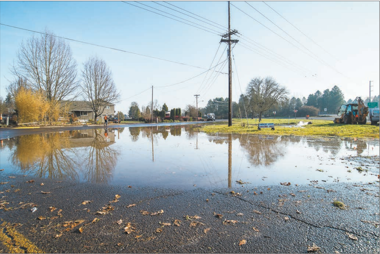
A large pool of water forms on Pacific Street after a 12-inch water main broke. Marcus Larson/News-Register
